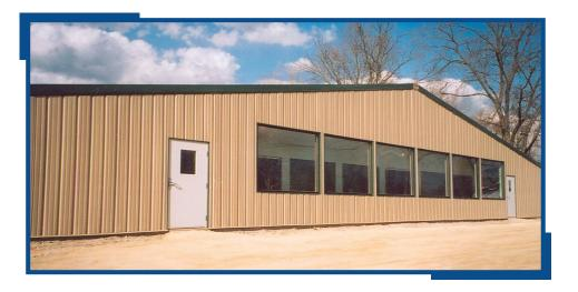
Glass storefronts are added in order to conform to the city's requirement on percentage of window openings.
