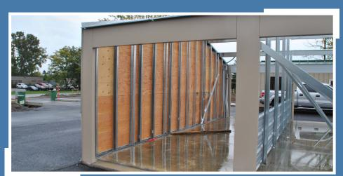
Trachte can provide steel studs to accommodate custom finishes to be applied by others. This project features studs with 16" OC spacing, in addition to the columns on 5' centers which support the roof structure.
