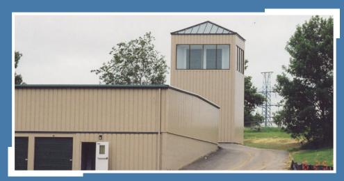
This tower is comprised completely of structural steel and helps to increase visibility of the site.
