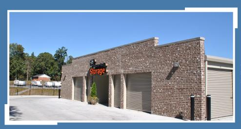
Nova Brick is featured on the endwall and two of the door jambs. The mortarless brick allows for a floating slab foundation.
