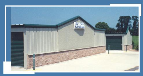
The center section of this building includes an efis material and a 4" wainscot of block.
