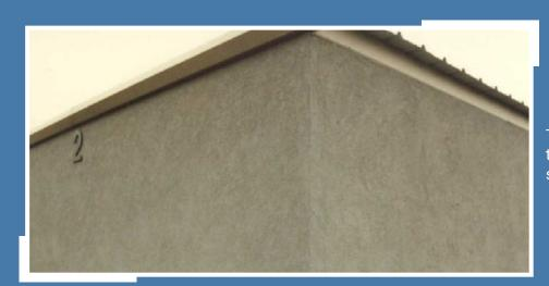
The EIFS material is typically installed on the sidewalls and endwalls that face the street.
