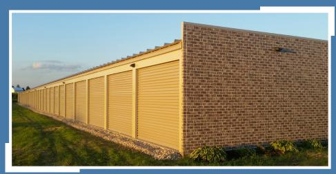
This building also has fake doors facing the street. The endwall is a parapet wall clad with Nichiha panel, which hides the lean to roof. Above the doors is the low side of the roof - water falls off the building into the tone below, which prevents mud from splashing back on to the building.
