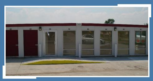
Glass fronts are utilized on the endwall of this building to convert the units into an office.
