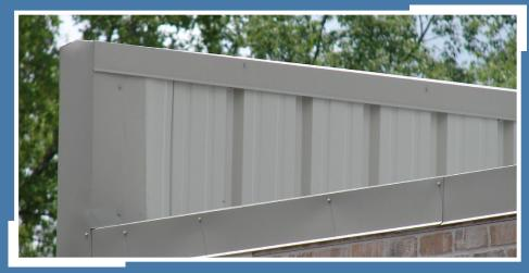
A parapet is a wall that extends beyond the roofline. Parapet walls may be used on endwalls or the high side of a lean-to structure. In some areas, they may necessitate the a roof designed to handle increased drift loads.
