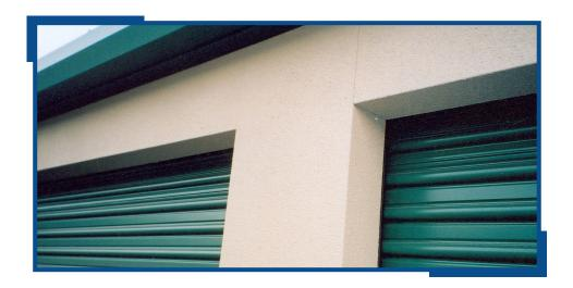
A Stuccoflex  $^{\text{\tiny M}}$  is applied to Trachte's door jambs and headers.
