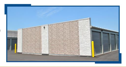
This building is accented by Nichiha's "Alexandia Buff" vintage brick panels. The cement board panels and mounting materials are provided by others and applied to Trachte's steel stud construction.
