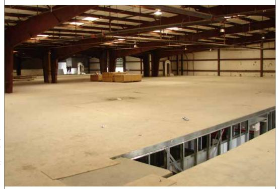
The second floor concrete is poured for this phased project. The lower level is rented first with the second level being developed in the future.
