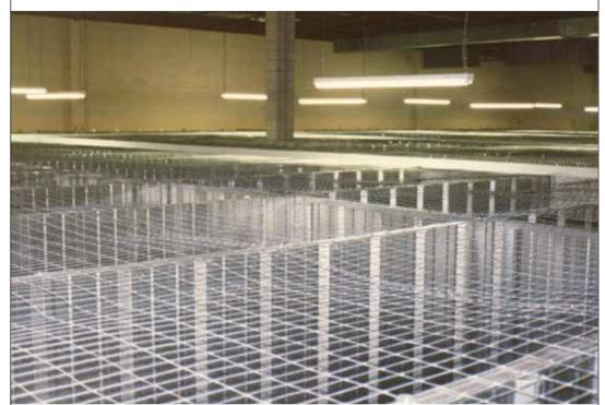
Wire mesh is installed over the corridor system. Special clips and screws are used to attach the wire to the structure.
