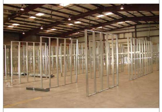
When a two story mezzanine is installed, the first level will feature load bearing stud walls to support the upper level. The open spaces between these wall sections will be hallways.
