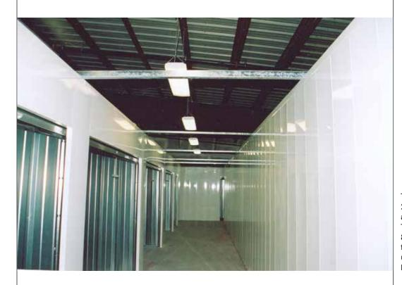
This corridor utilizes 24-gauge flush panel along the entire wall. The complete system is 8'6" high, which allows for roll-up doors on all units. The ceiling was left open over the halls.
