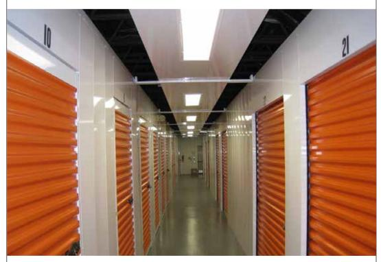
Swing doors are used for the smaller units while roll-ups are used for the larger units. Swing doors are easier to ship so they are recommended for units going via sea container because they take up less space.
