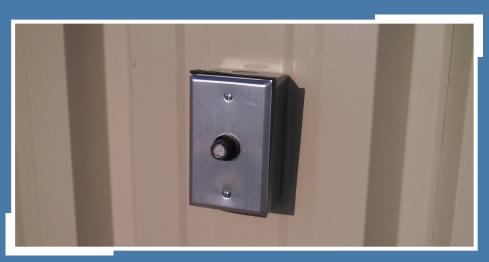
Exterior lights should be controlled by a master photo cell rather than individual sensors on each light.
