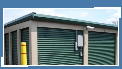
If the building has a false door, the electrical panel may be attached directly to it.
