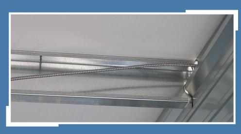
The electrical conduit should be installed following the purlin.
