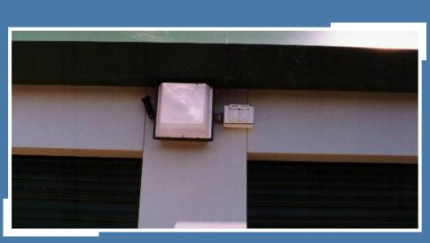
At least one exterior outlet should be installed on every building for maintenance puposes.
