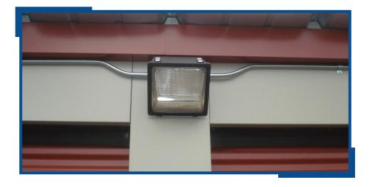
This exterior light has the conduit running on the outside of the building. This application is not recommended.
