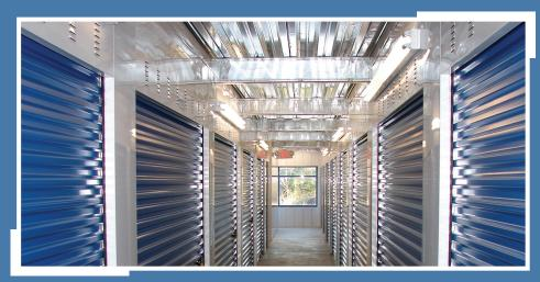
The lights can be attached directly to the corridor. However, this lighting is not recommended because the light will only shine into one side of the corridor.
