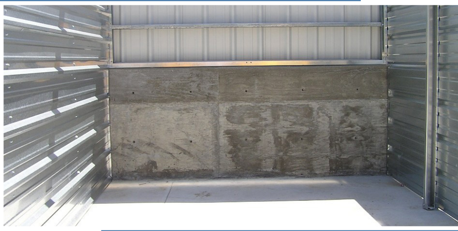
An inside view of the retaining wall.
