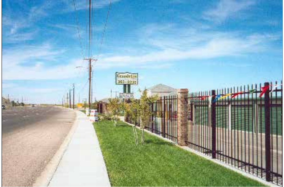
A brick column every 40' accents the aluminum fencing.
