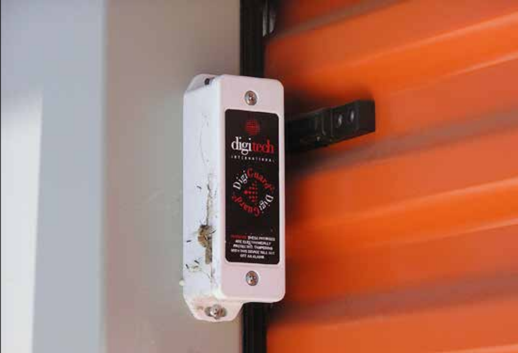
Exterior-mounted radio frequency door alarms can be added to an existing site.
