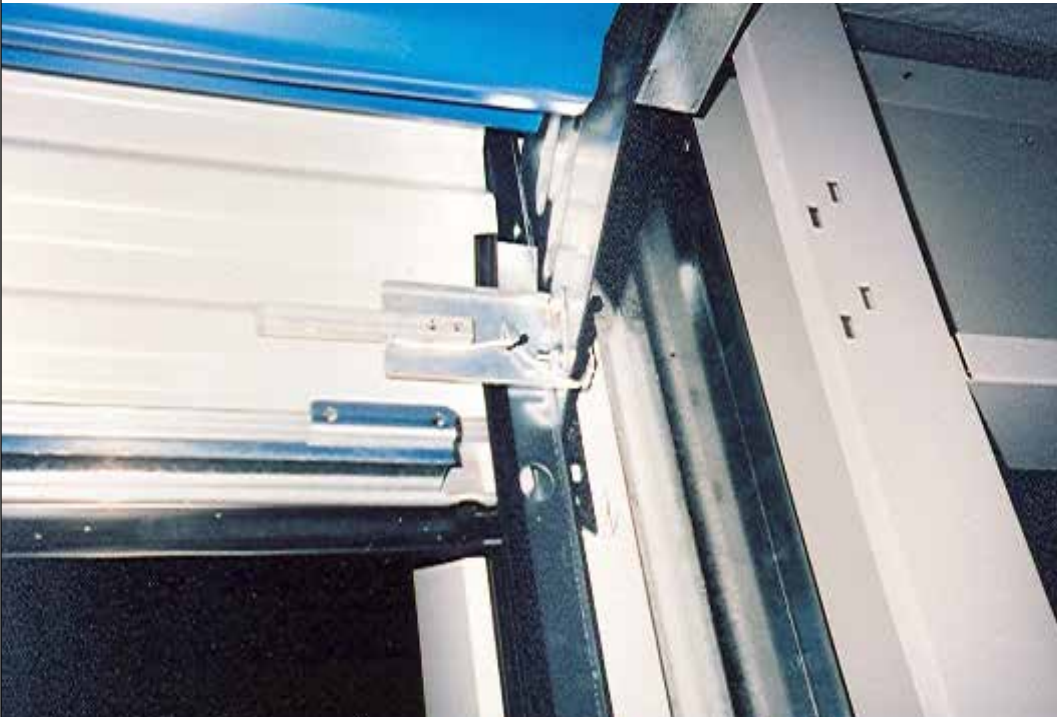
Hard-wired door alarms, such as the Track-It system, attach directly to the doorstop.
