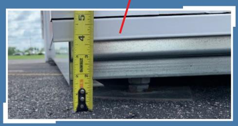
On the high side you will have the leveling feet screwed in completely which makes the step up roughly 6".
