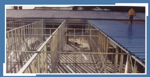
After the concrete floor is poured, a galvanized stud wall is assembled and a 20-gauge metal floor deck is installed on top of the stud wall.
