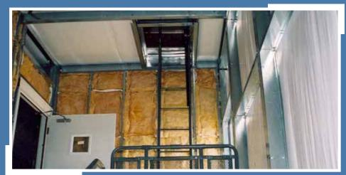
For a three story building a roof hatch with ladder is required to access the roof.
