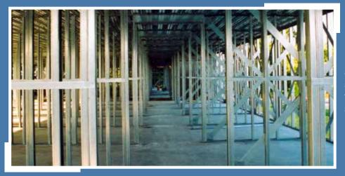
If the building has an interior corridor, a stud wall header system is used to support the floor load. A 20-gauge metal floor deck is then installed on top the stud wall.
