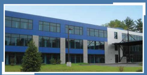
Trachte buildings may be highly customized. Built by a Varco Pruden dealer using Trachte building structure and interior, this structure is clad with architectural panels and glass curtain walls.
