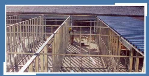
A galvanized stud wall is assembled and a 20-gauge metal floor deck is installed on top of the stud wall.
