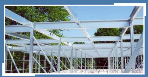
The second floor structure is installed on the cured slab.
