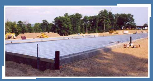
The long-span metal floor deck is ready to pour.
