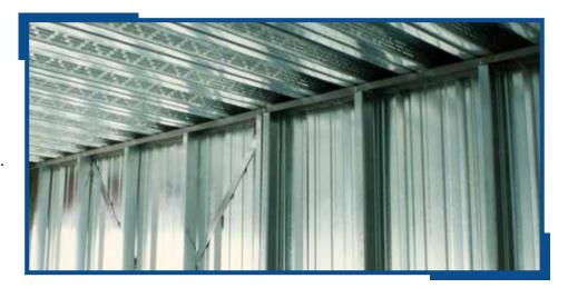
Galvanized stud wall with a 20-gauge floor deck to accept concrete by others.
