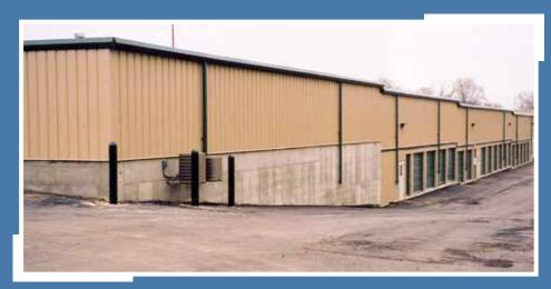
This site does not allow access on both sides of the building until the drive is level with each unit. The city only allowed a 7% grade so it took more driveway to get to the 10'8" grade change.
