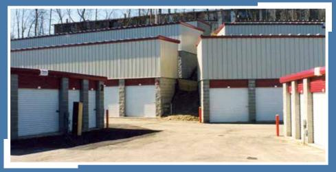
This site was maximized by building three two-stories into a hill to overcome its 30' change in elevation.
