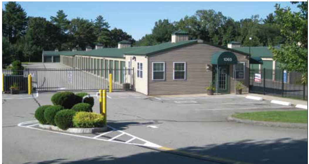
The 30' x 30' x 9'4" office has a 3:12 pitch. Horizontal siding and cupolas add visual interest to the office. The awning displays the street number and provides a nice entry to the office.
