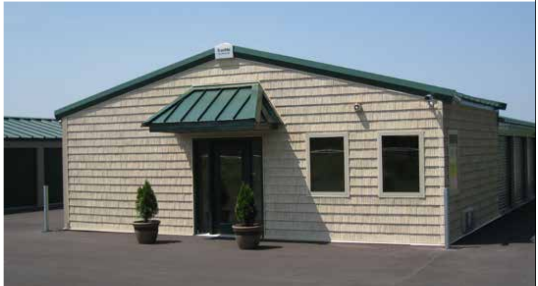
The 30' x 30' x 10'4" office has a 3:12 pitch. A shake siding is used on the exterior. Trachte supplied the metal awning over the door.
