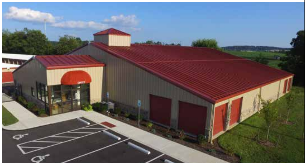
This unique office design features an offset ridge and is adjacent to a wide climate controlled storage building. The storage building features false doors to help communicate the purpose of the building.
