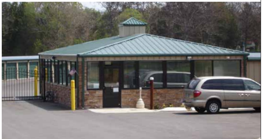
The 30' x 30' hipped office combines a roof with cupola with a brick wainscot.
