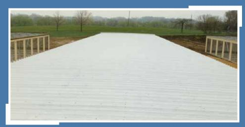
Trachte's galvalume R-panel roof sheets span from eave to eave on low-pitched buildings up to 40' wide, eliminating additional costs for ridge caps and installation.
