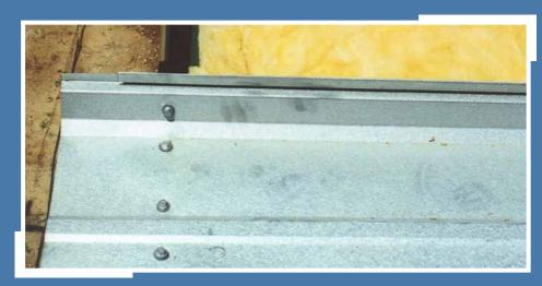
The 2' standing seam roof panels are fastened to the exterior eave angle, tape caulk, and metal closures.
