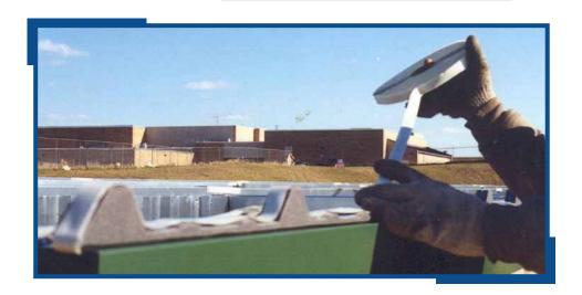
3' foam closures are installed with Presstite tape caulk above and below the closures.
