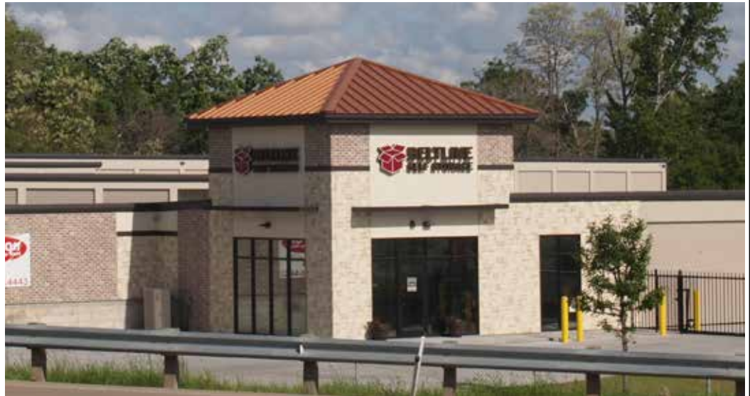
The sign at Beltline Storage was custom made and includes a logo.
