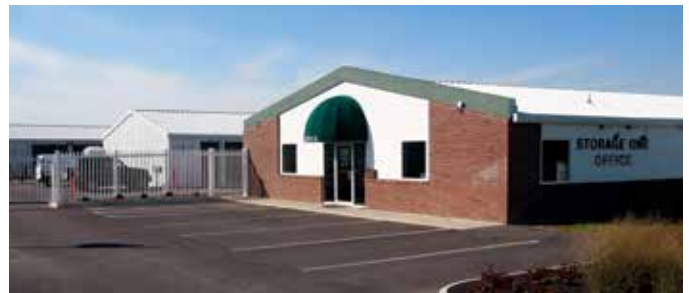
Brick and stucco parapet endwalls are the signature features for this client's properties
