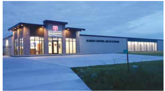
Exterior facade with fiber cement panels and insulated steel salewich panels (supplied by others)
