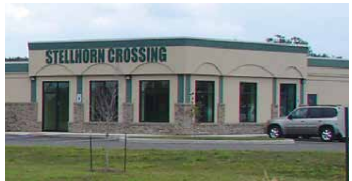
Brick wainscoting and glass entry door
