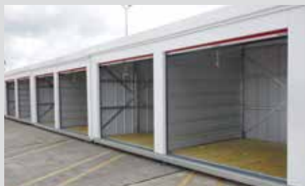
Wood floor inside unit
