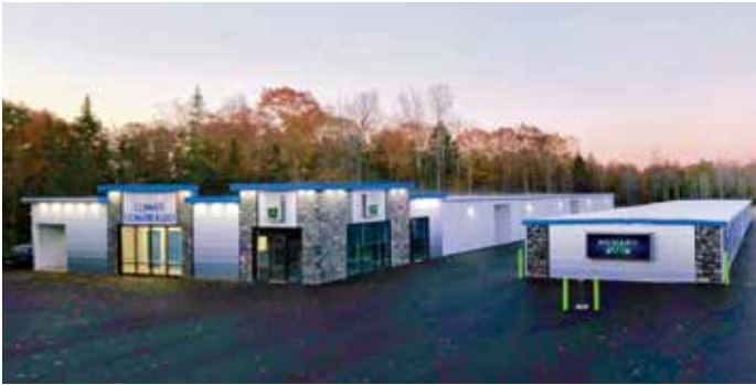
Varied height parapet with stone front, windows and custom facade
