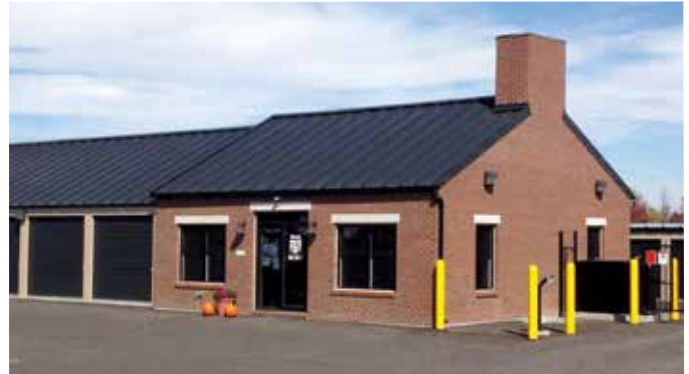
A brick exterior wraps the Trachte structure of this office
