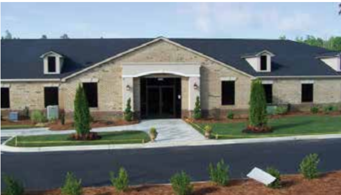
Office with brick facade, dormers, false windows, and shingle roof
