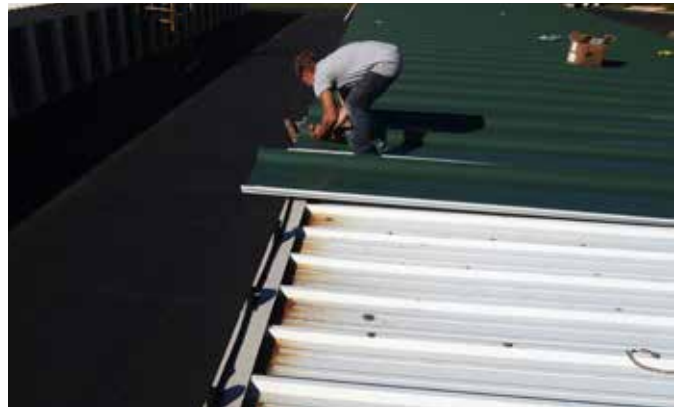
Overlaying new roof panels over existing roof.
