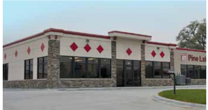
Parapet walls, stucco, masonry finishes, and commercial windows create a retail storefront feel on this insulated structure.
