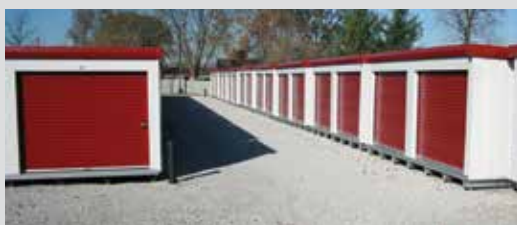
Entire site comprised of modular units
