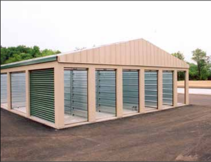
16. The finished end closet.
