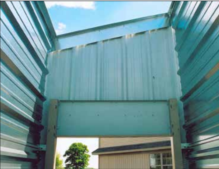
17. An inside view of an end closet 5' x 10' unit.
