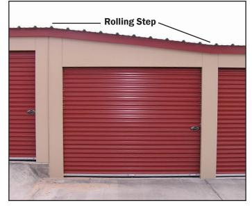
h. An alternate way to accommodate a roof step is to use a rolling step. This design can be used for steps up to 12" in height. Please contact the Trachte Regional Manager for limitations and other information.
