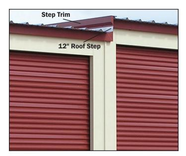
g. When there is a change in foundation grade, building steps will be required. For steps 12" or less, the step trim color will be determined by the rake trim color and the starter strip color will be determined by the roof color. For steps greater than 12", additional rake trim and A-Type panel will be included at step. The starter strip color will be determined by roof color. Contact a Trachte Regional Manager if you have any questions about building steps.
