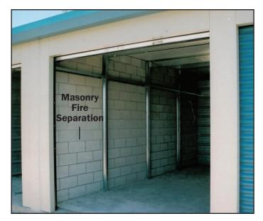
k. If an interior masonry fire separation is required, the structural framing includes exterior trim pieces to cover the fire separation.
