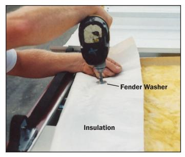
n. 3/4" vinyl-faced insulation is recommended to prevent condensation on the roof. The insulation is installed using fender washers.
