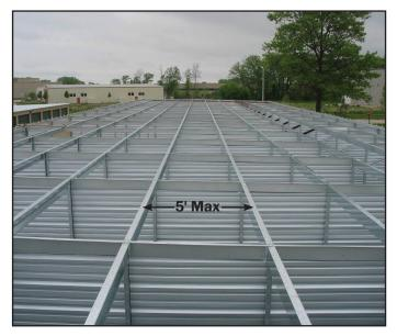
The interior structure has 5' purlin spacing standard, in some high snow load areas closer purlin spacing may be required.
