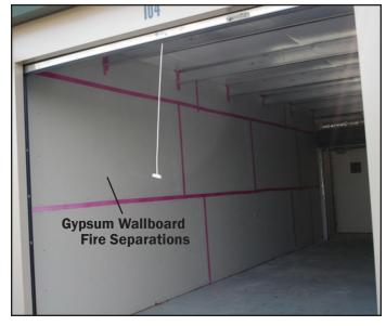
i. For interior fire separations, gypsum wallboard is installed over stud wall and taped. Number of sheets on each side of stud wall will vary based on fire rating needed.
