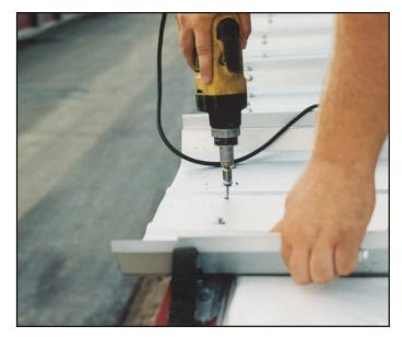
p. The standing seam roof need only be screwed down at the eave. This prevents having exposed screws across the roof sheets, minimizing the potential for roof leaks. Trachte highly recommends the standing seam roof, which features 2' wide snap together panels.
