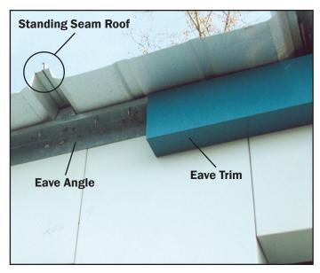
p. The screws at the eave are located outside the building to prevent roof leaks. The eave trim covers the eave angle and roof screws for a clean, finished look. This feature is standard on all Trachte buildings.
