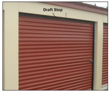
Header draft stops are used to seal the top of the door to minimize dust, dirt, and blowing snow from entering the unit. Draft stops may be added to a proposal or may be purchased at a later date.
