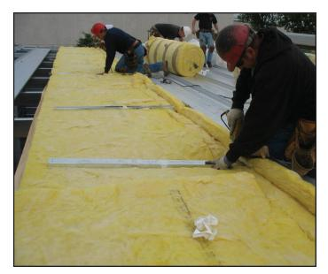
n. Trachte offers up to an R-38 (12") roof insulation. Shown above is a R-32 (10") roof insulation using R-5 thermal blocks. Contact a Trachte Regional Manager about meeting energy codes.
