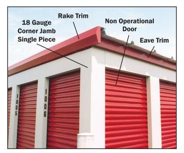
f. Rake trim covers the end of the building while eave trim covers the side. Both rake and eave trims are used to accent the building and are normally the same color as the doors.
