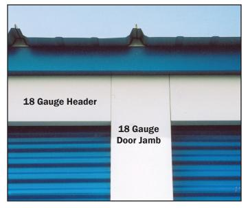
Door jambs and headers are constructed of prefinished 18 gauge material, which is 2-1/2 times thicker than the industry standard 26 gauge material. Jambs and headers feature no exterior fasteners giving a clean, finished look.
