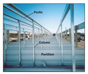
b. The interior structure features pre-punched columns and purlins for bolt together connections to simplify installation. The entire structure is zinc coated to inhibit rust.
