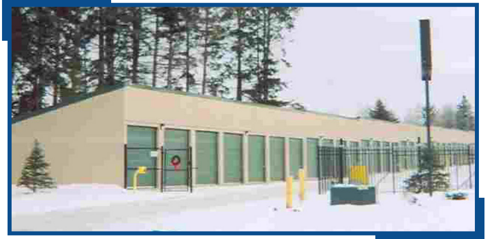
A 3":12" pitch, lean-to building with the doors on the high side.
