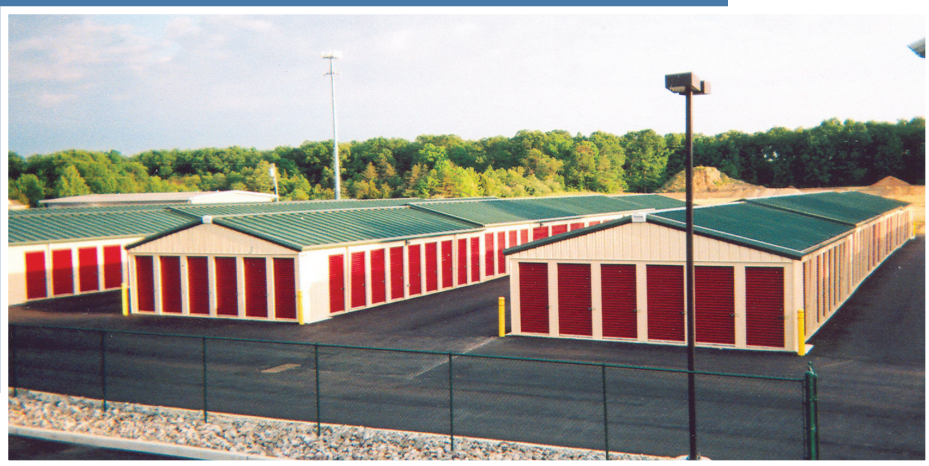
View of the entire site.
