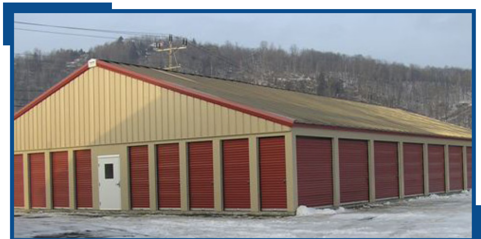
60' wide, 4":12" pitch, Classic Beige building with Cedar Red doors, roof, and trim.
