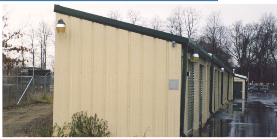
15' wide, 3":12" pitch building with doors on the low side.
