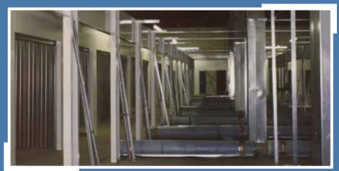
20-gauge Bright White corridor units are assembled following Trachte's erection guide. The door jambs are installed to an angle framework and then the partition is attached.
