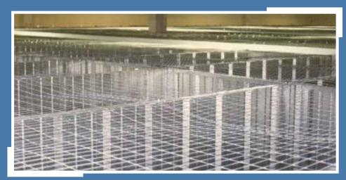
Wire mesh is installed over the corridor system. Special clips and screws are used to attach the wire to the structure.
