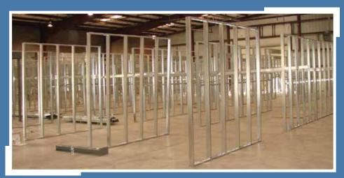
When a two story mezzanine is installed, the first level will feature load bearing stud walls to support the upper level. The open spaces between these wall sections will be hallways.
