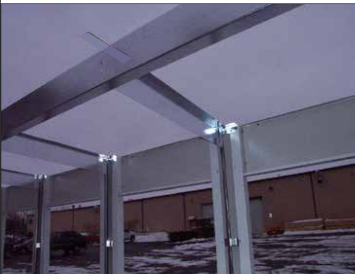
90. Install all the rake angles (if purchased) between the purlins. The rake angle fills the void at the top of the partition wall. Rake angles are only needed where partition panel is planned. All rake angles must be installed before roofing.
