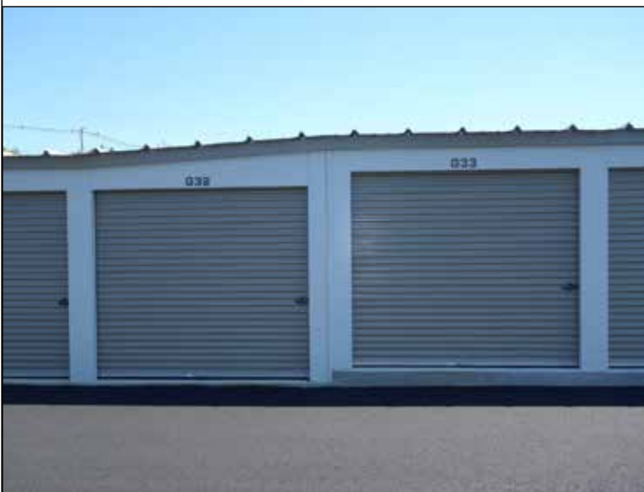
200. Here is a view of the finished unit.
