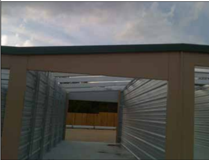
198. A special header is used and the trim follows the slope as shown.
