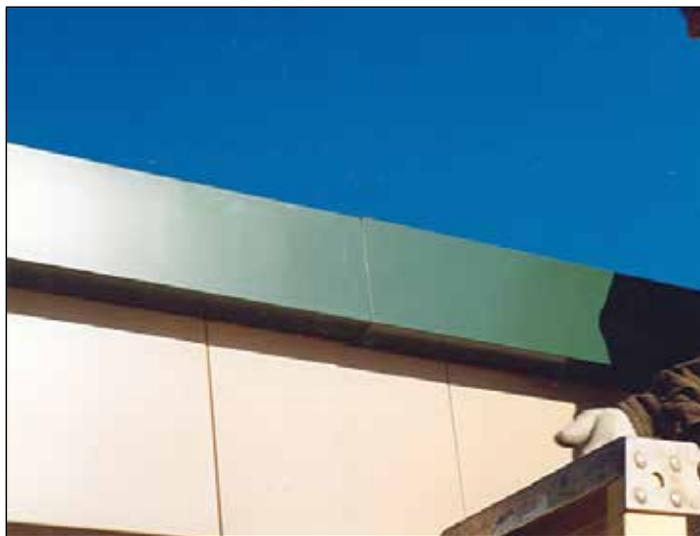
TEMPORARILY FASTEN EAVE TRIM WITH 2-SCREWS. PLACE SCREWS WITH CONSIDERATION AS TO WHERE ROOF CLOSURES AND FASTENERS WILL BE INSTALLED LATER. BACK SCREW THE BOTTOM OF THE TRIM TO CLOSE THE GAPS. BE SURE TO HIT THE LIP OF THE TRIM.
